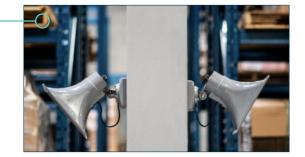
to or from Yealink phones via multicast. Multicast groups are easy to configure as long as Algo endpoints and Yealink phones are on the same LAN segment. Any device can send or receive audio from other devices within a group. Algo IP Speakers for voice paging feature wideband audio to deliver clear audible communication for speech intelligibility and background music.
